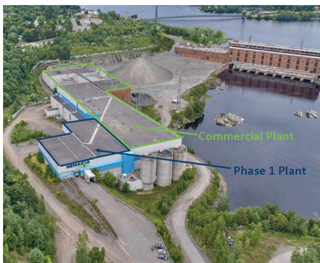
Abb. 19 – Nemaska Hydroplant Quelle: Nemaska Lithium Inc.
